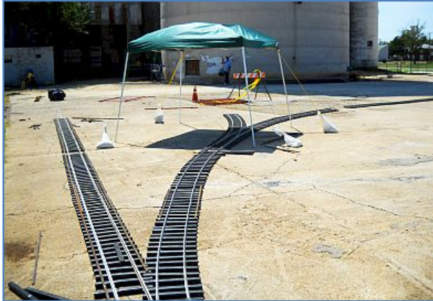
Shade was provided for the track work.
