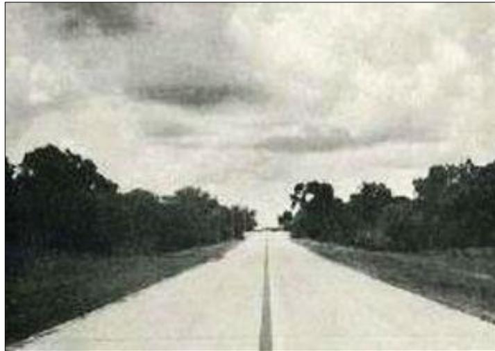
**Center Strips painted on curves, hills and bridges divided the pavement into two lanes for safety.**
